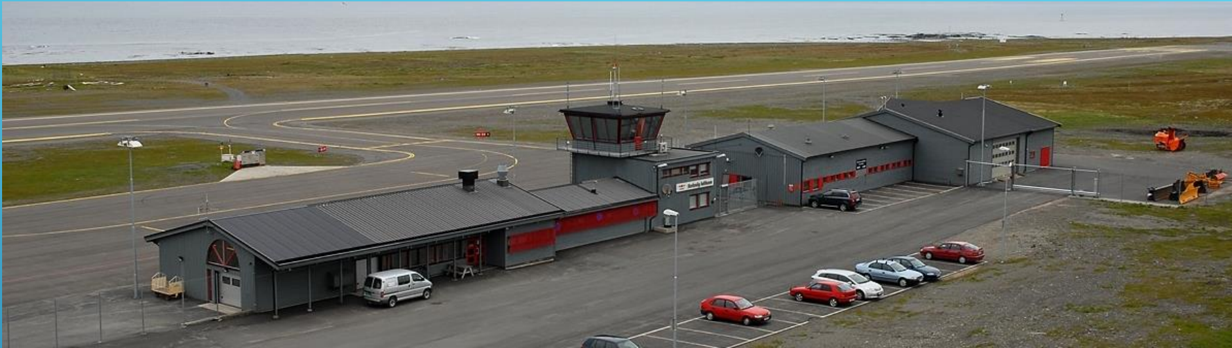
ENBV – Berlevåg airport. Photo: Avinor
